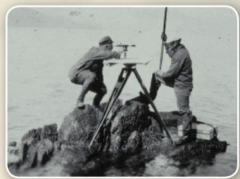
Coast and Geodetic Survey crew uses a plane table to map shoreline in Southeast Alaska circa 1921.
